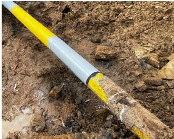
Photo 2. May 2023 6-Foot Section Replacement
